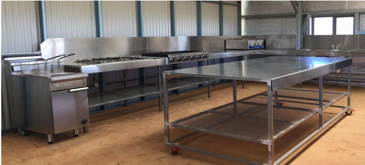
Jundah Recreation Reserve kitchen upgrade
