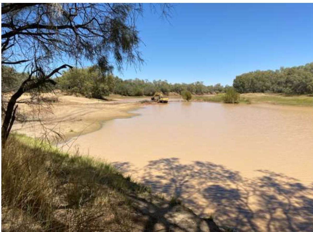
Image of works at McPhellamy's crossing, Cooper's Creek
